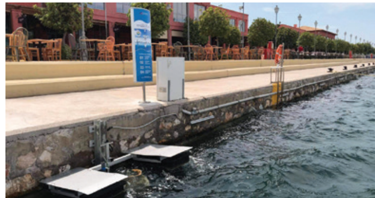
Seabin presents an innovative solution for the removal of plastics from a marine environment
